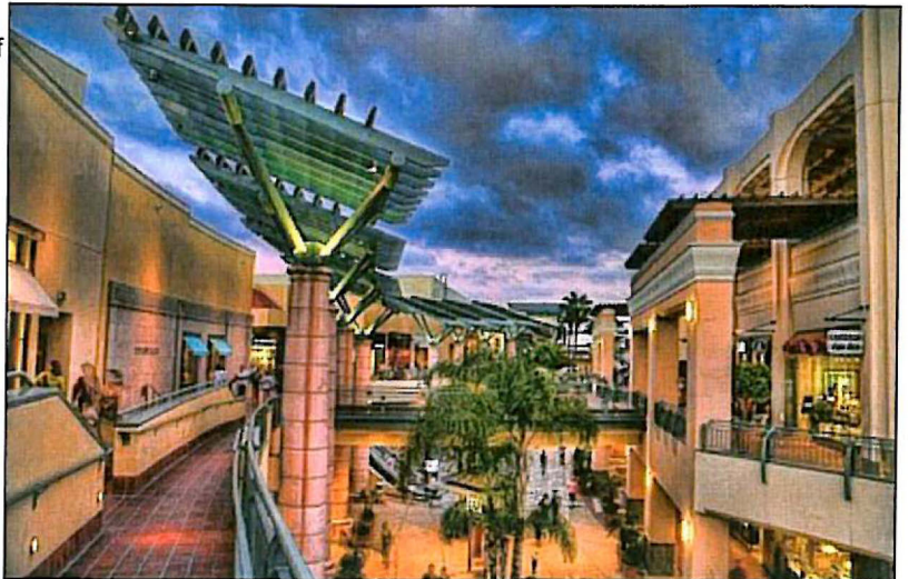
One of ELEN's recent projects was a Lighting System Upgrade at Fashion Valley Mall.
